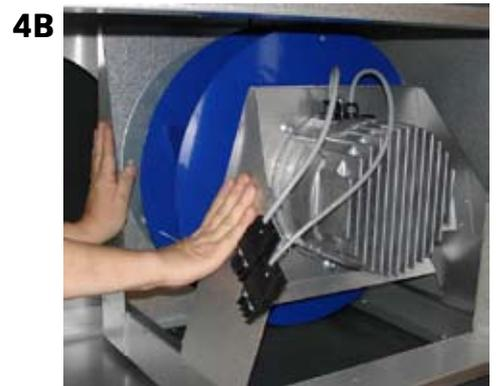
**Step 1:** When disassembling the connectors (1) and the rubber tubes (2B/3B) each unit module must first be disconnected (fig. 3 page 4). Unscrew the lid which the connectors enter and pull the connectors through the whole (2A/2B).
